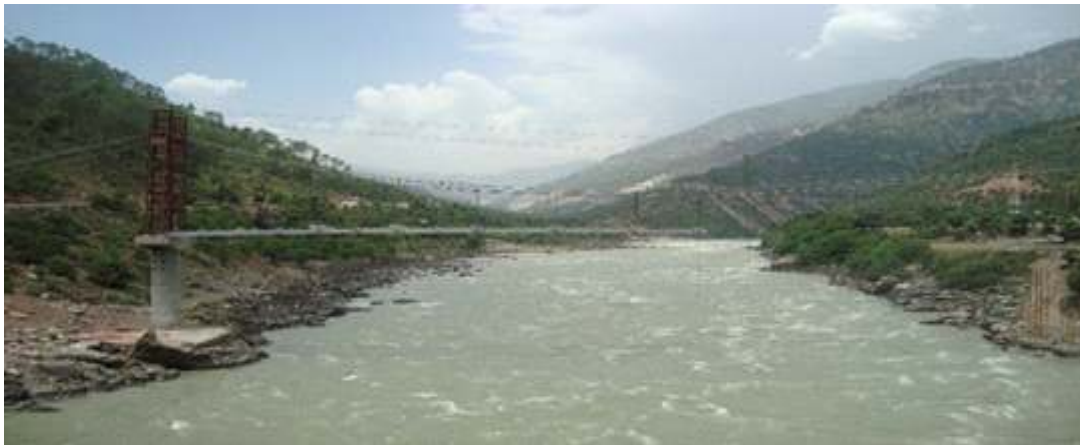
Picture 5: Launching of Steel Truss of Bridge Through cables
