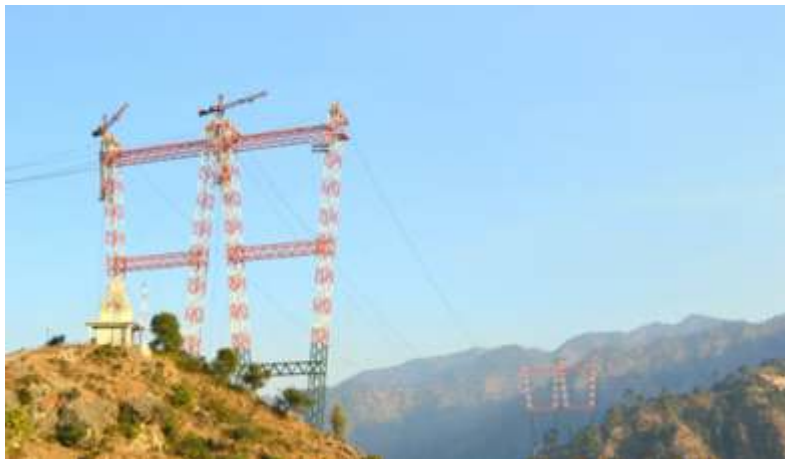
Picture 1. The cable way for Chenab bridge
