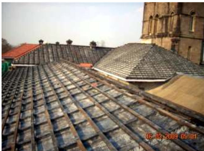
Wooden trusses of roof after repairs
