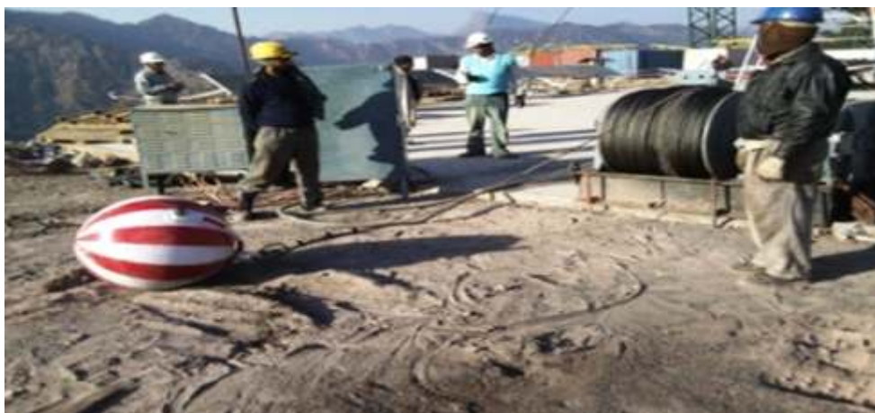
Picture 2: The steel ball for crossing the cables
