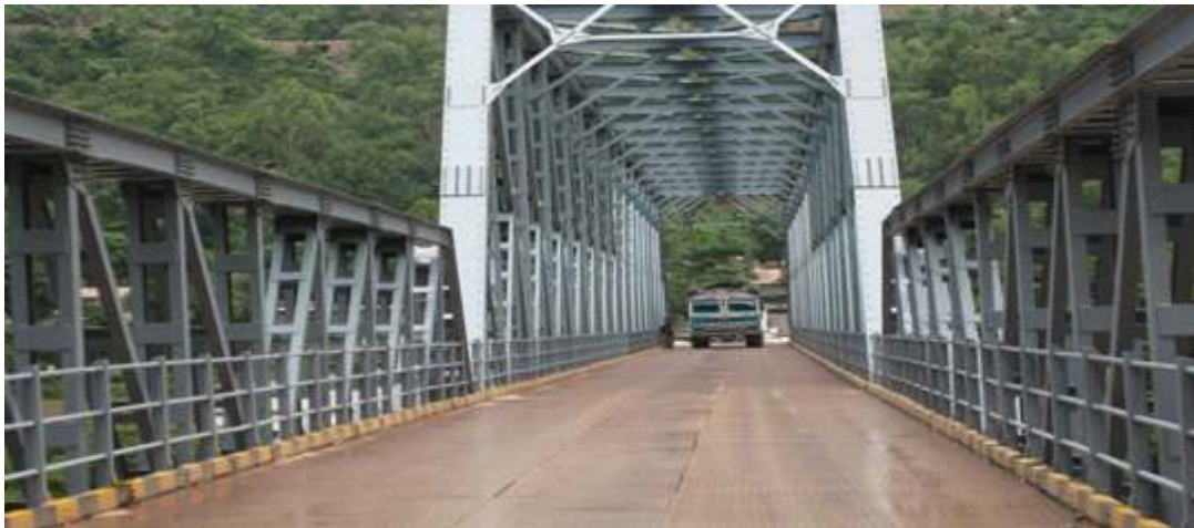
Picture 6: Completed Bridge Opened for Heavy Axle Load Traffic
