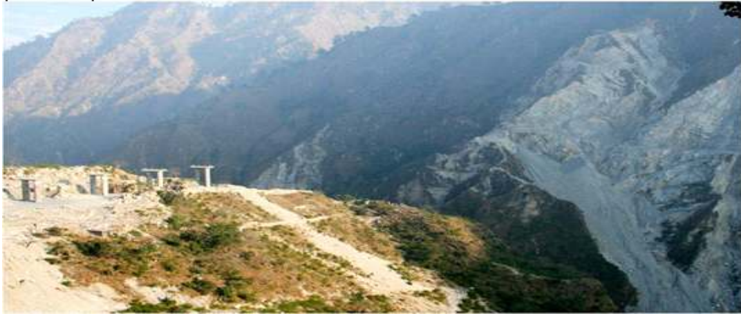
Picture 3: Anjikhad Site with Difficult Geology
